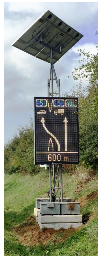
Photo 1: PMV à LED programmable
